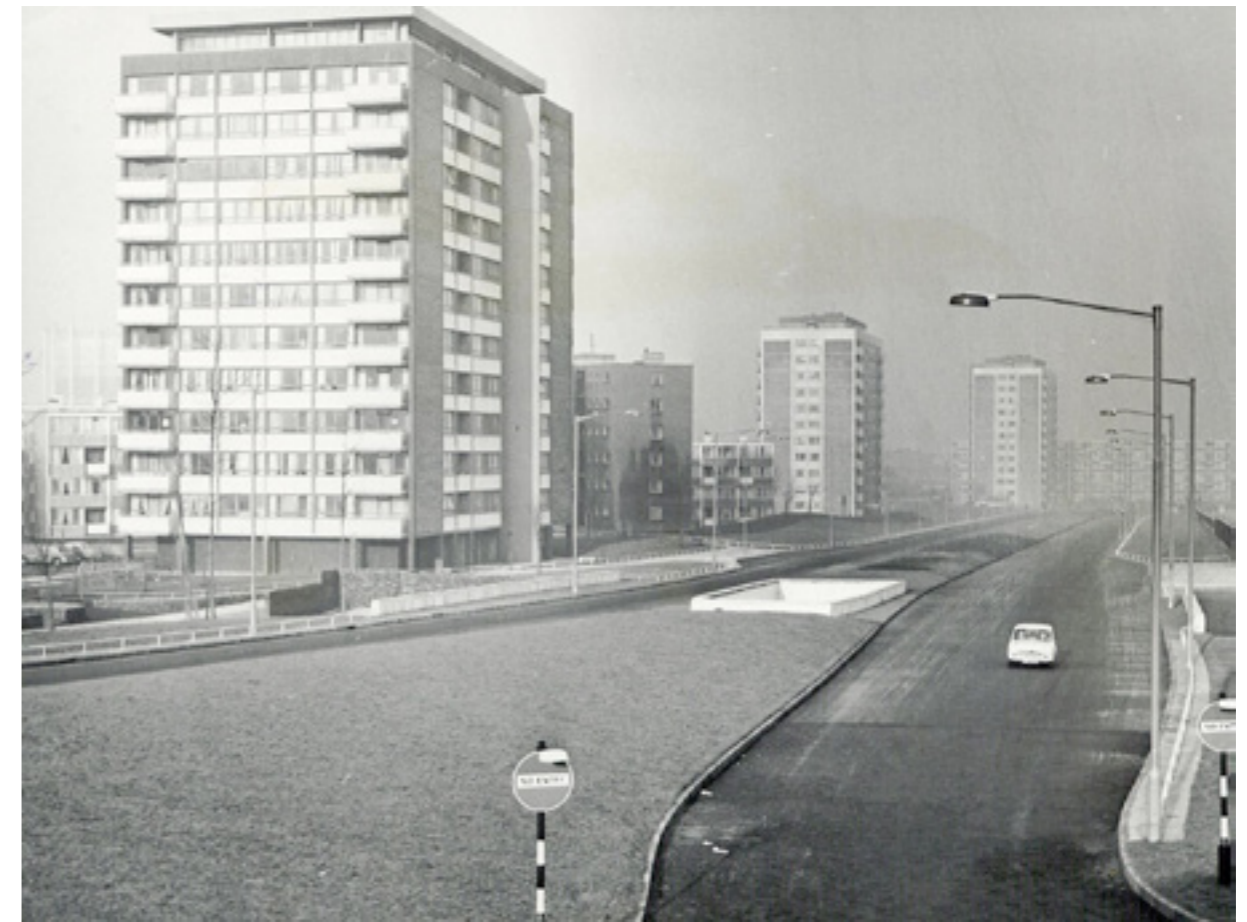
Tower blocks in Nechells, 1963. © Birmingham Mail.
